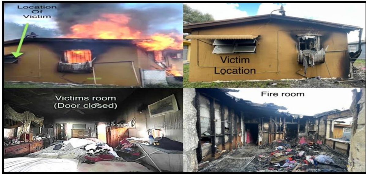
(FIGURE 2) THESE PHOTOGRAPHS ARE OF THE BATT 5 GRAB MENTIONED ABOVE. THEY SHOWCASE THE IMPRESSIVE CAPACITY OF A SIMPLE RESIDENTIAL INTERIOR DOOR TO EFFICIENTLY WITHSTAND SMOKE AND FIRE. BY MAINTAINING DISCIPLINE AND TAKING ADVANTAGE OF THIS POTENTIAL, WE EMPOWER OURSELVES TO REACH OUR HIGHEST LEVEL OF PERFORMANCE, AS R202 DID ON THIS FIRE RESULTING IN A SAVED LIFE.
